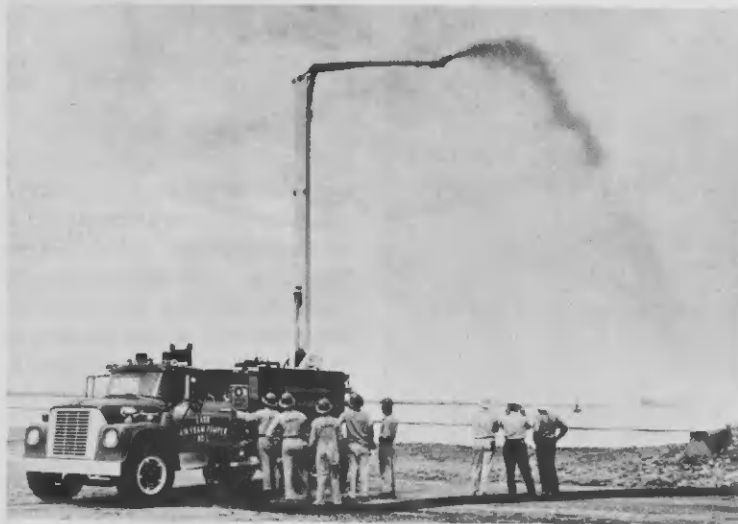
New feature is articulated boom, shown here in action.
